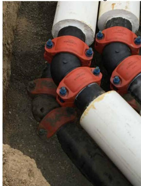
Without *Victaulic*'s coupling technology, more than 75 percent additional labor would have been needed for the installation of the HDPE piping systems.
