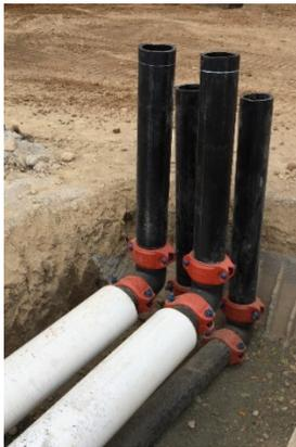
Insulated and non-insulated HDPE pipe is joined using *Victaulic* fittings and couplings in both horizontal and vertical orientations for hydronic hot and cold water distribution at the new Four Seasons Napa Valley Resort in California.
