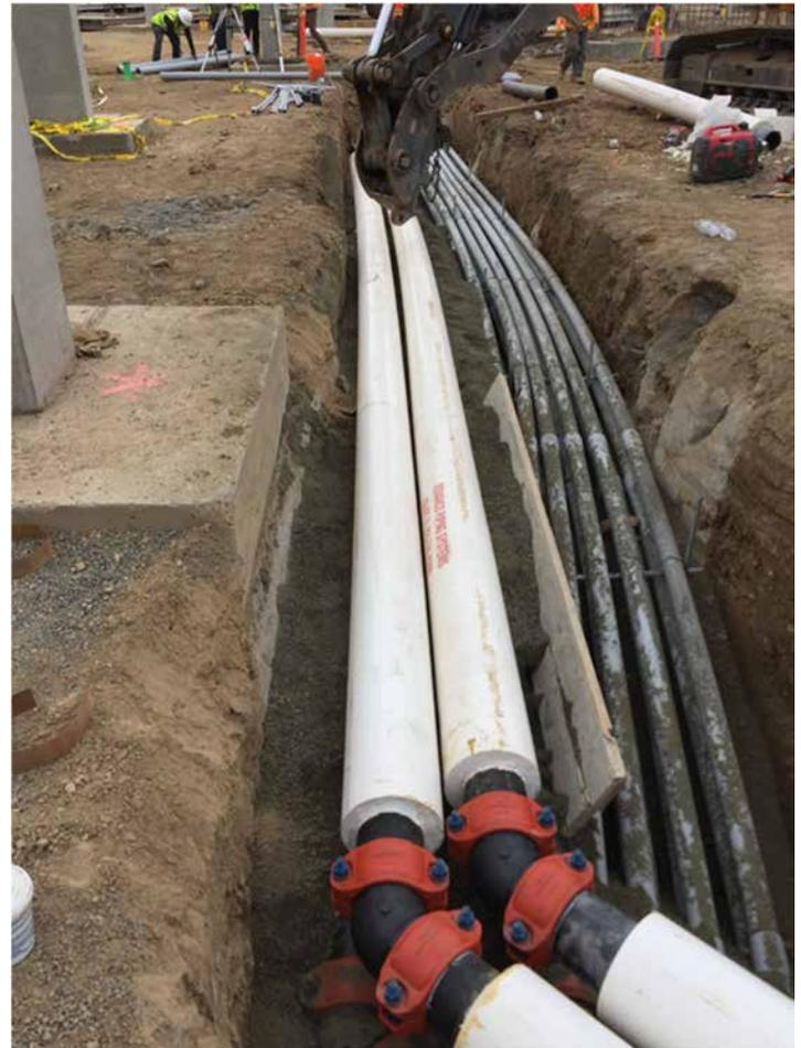
The insulated and non-insulated HDPE pipe is joined to *Victaulic* HDPE fittings using *Victaulic* Style 905 Couplings. A fully restrained system, *Victaulic* fittings and couplings are designed to be buried.
